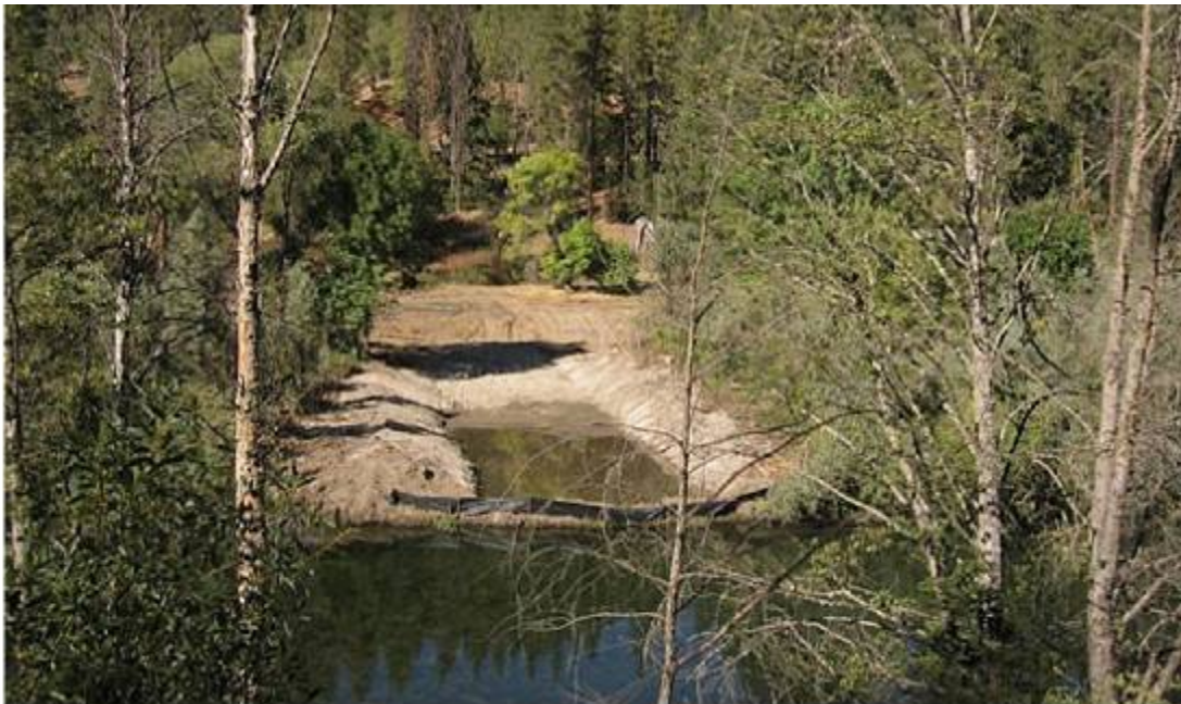
Berm notching at Vitzhum Gulch. Photo by the Trinity River Restoration Program
